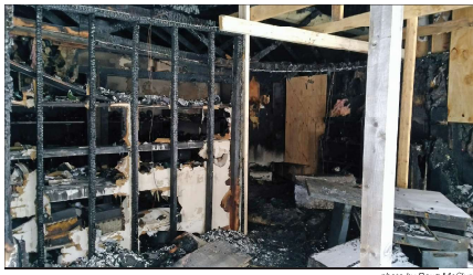
Photo by Doug McClure The studio of the Vermont Glass Workshop on Mainville Road caught fire on December 29. Co-owner Harry Besetti said the fire was caused by a propane tank that was not properly secured. Friends are helping him raise money to assist him in rebuilding their business.
