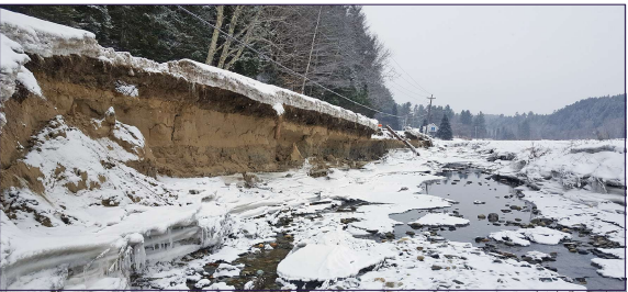
North Wolcott Road washed out as a result of flooding caused by ice jams. The road surface is at upper left; telephone poles lean precariously over the roadway. The view is from the river; the exposed dirt is where the flood undermined and collapsed part of the road.
