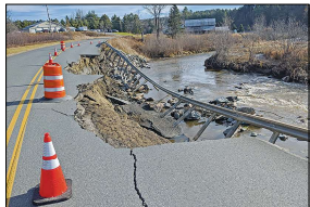
photos by Enoch McGraw At the Craftsbury end of North Wolcott/Wild Branch Road, half of the road was washed over by the Wild Branch during the Halloween storm.
