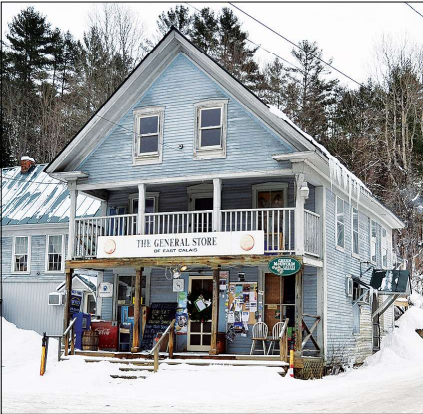
The East Calais General Store is being torn down. It has been closed since Christmas. A new community group called The East Calais Community Trust is working to purchase and renovate the building and get a new store in the space.
