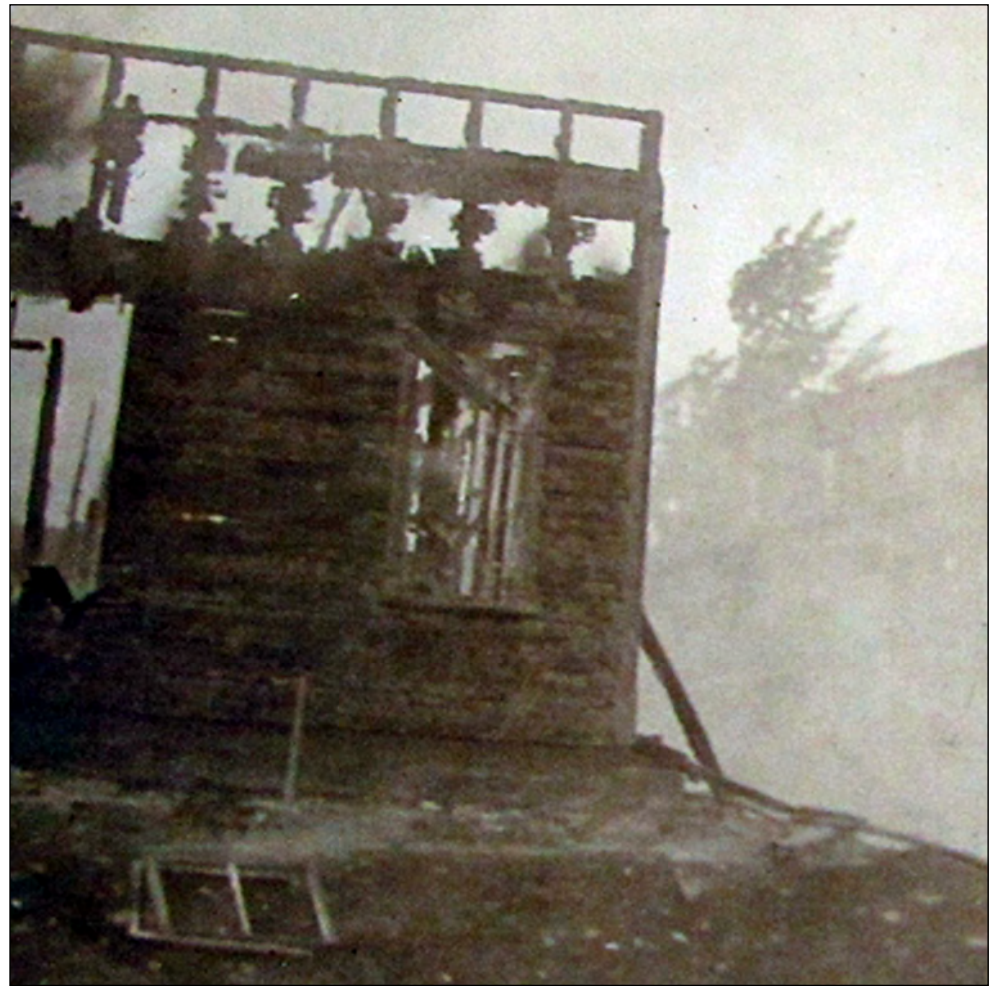
photo by Clifford Daniels, Craftsbury Historical Society archives A burned-out shell was all that remained of the Clyde Gilbert family's home on Cemetery Road in Craftsbury Village after a devastating fire on July 12, 1931. The third floor of the Taylor Building is visible in the background through the smoke.
