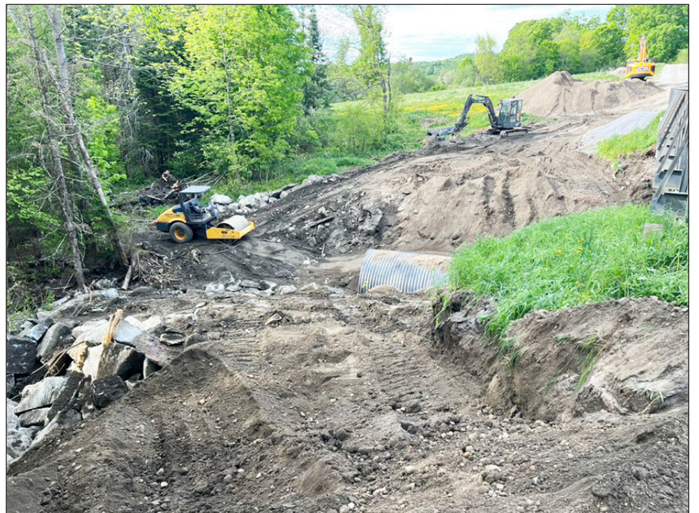
Work continues to replace a culvert under Menard Road in this photo taken Wednesday evening, May 28 photo by Sid Griggs
