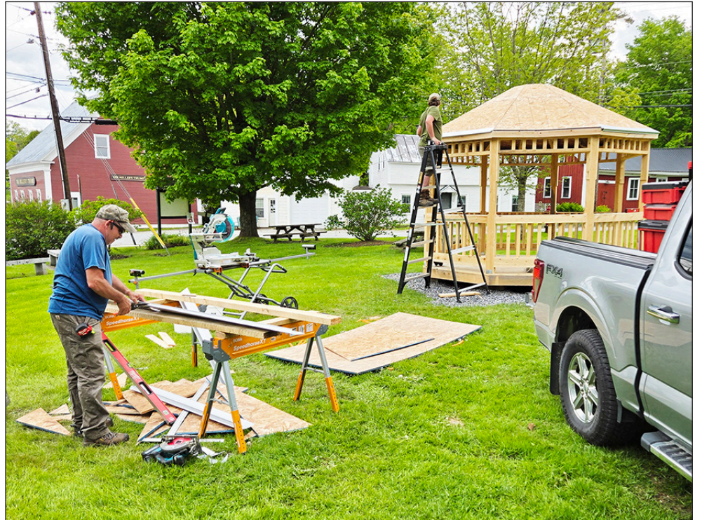
Corbin LaPierre stands on a ladder to add drip edging to the new Greensboro Gazebo’s roof in the park across from Willey’s Store, the afternoon of June 2, while his father Mike cuts the next piece to size. photo by Paul Fixx
