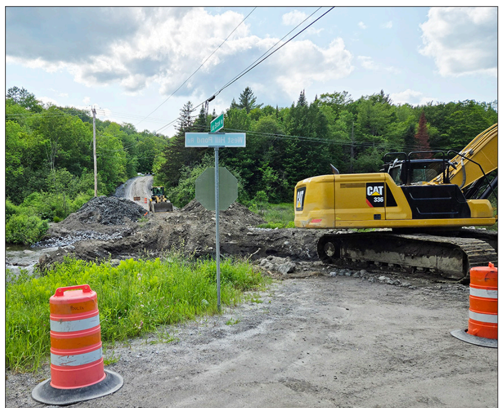
Jug Brook Road in Cabot is closed for construction at its intersection with W. Hill Pond Road in Cabot, Saturday, June 14. The upper and lower culverts are being upgraded and a bypass has been installed at the lower culvert excavation to dry out the area prior to installation of concrete footers, stem walls and box culverts.
