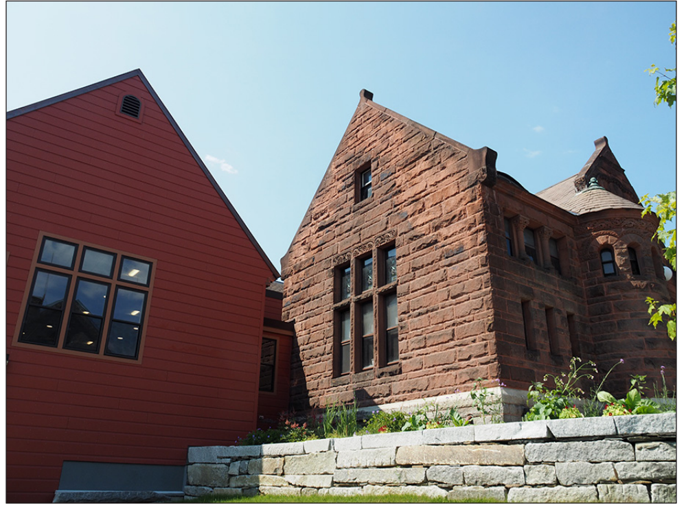
The Jeudevine Library's new addition to the left contrasts with the original library built in 1896. photo by Alex Strand
