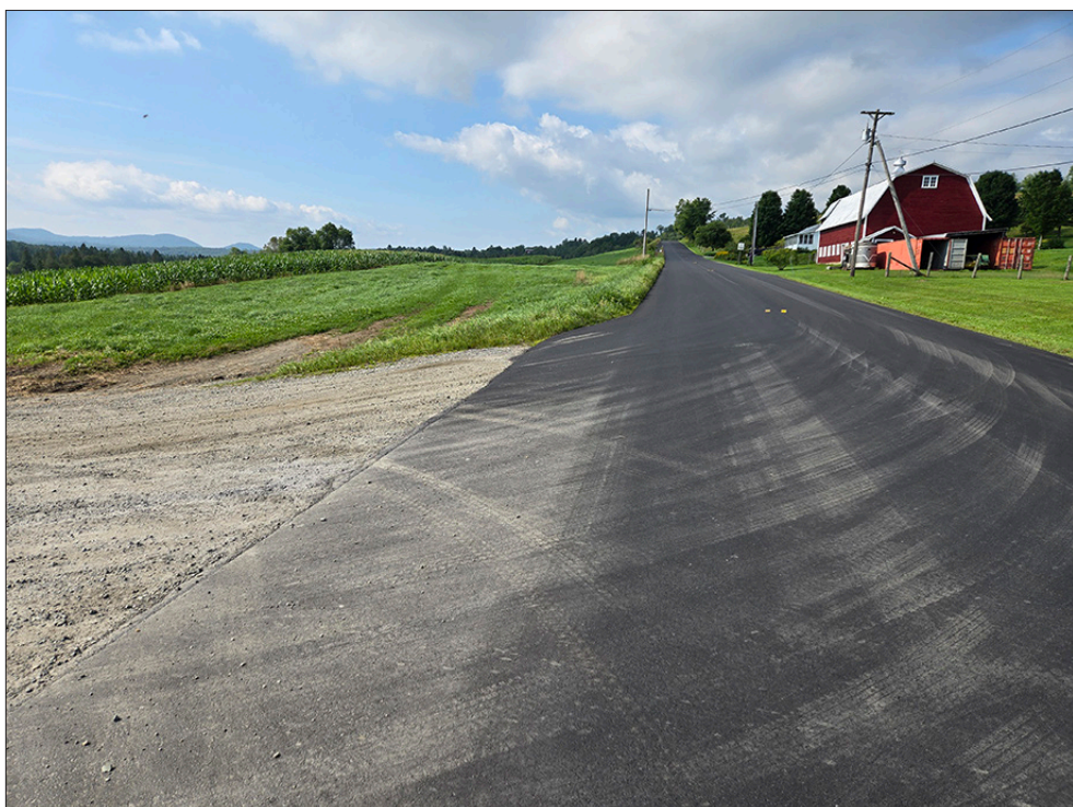
Paving of Center Road between Hardwick and Greensboro was completed Monday, after a break for rain last Friday, in this view toward Hardwick at Hardwick Farms Road in Hardwick Center. All-in-all, the work took Pike Industries five work days and only the center line, now temporarily marked, remains to be painted. photo by Paul Fixx
