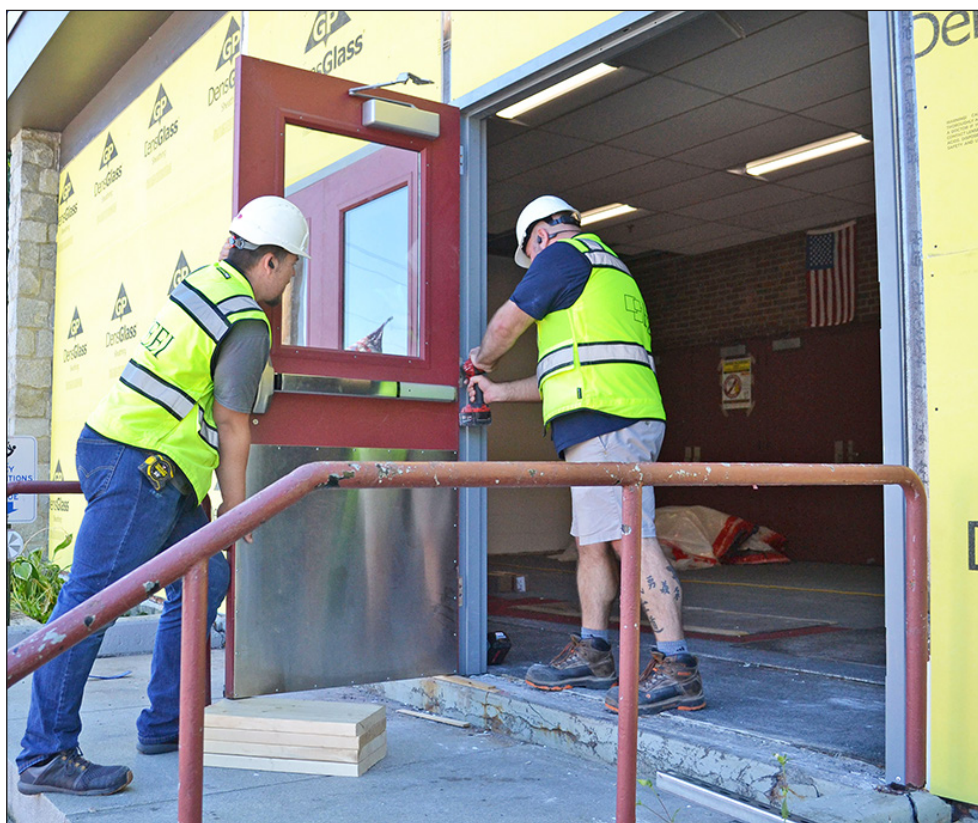
Energy Efficient Investments site supervisor Brian Depinto (left) and project coordinator Luke Aither (right) rehang the old doors to the Hardwick Elementary gym lobby, August 21. New support beams were welded in place, and temporary walls were installed, until the new doors and windows are delivered. photo by Vanessa Fournier
