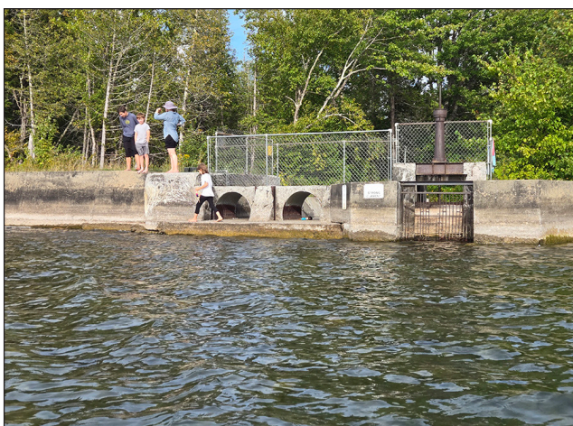
Measurements on Labor Day, Monday show the Caspian Lake level at 11 inches below the spillway. The average September 1 water level over the past 8 years has been 12.2 inches higher, confirming anecdotal reports that the lake is at an historic low. photo by Paul Fixx
