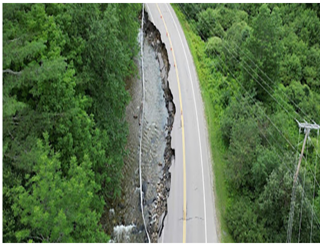
The flooding in 2024 washed out roads and bridges across Vermont.
