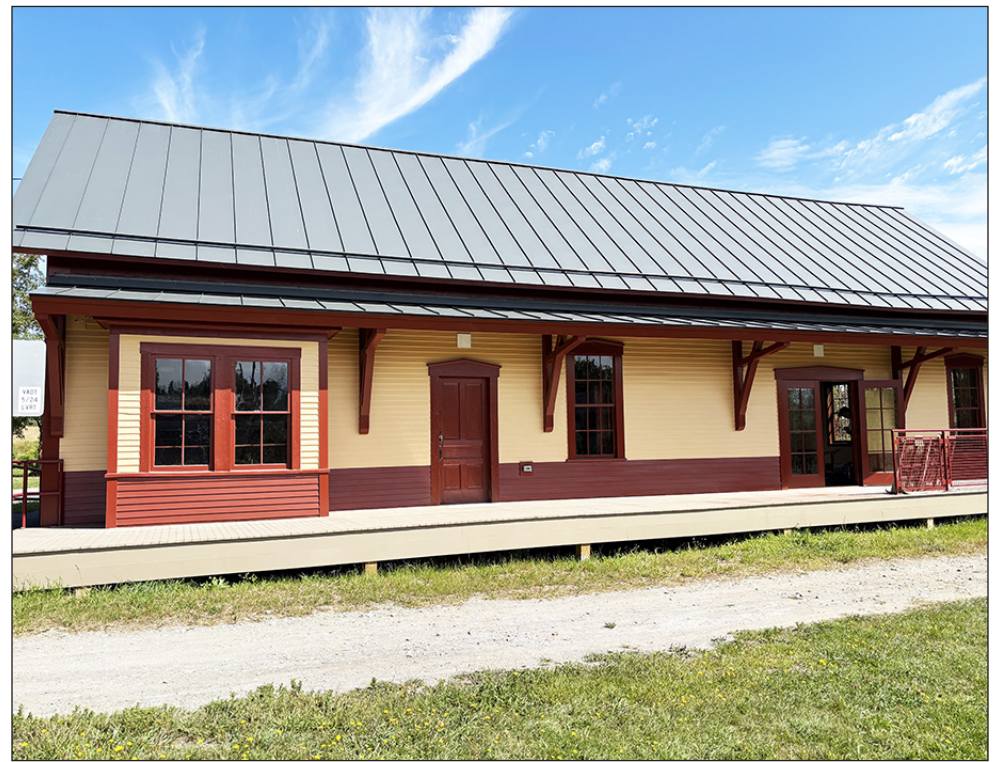
The renovated train station in Danville on the Lamoille Valley Rail Trail will be featured at an open house on September 18. courtesy photo
