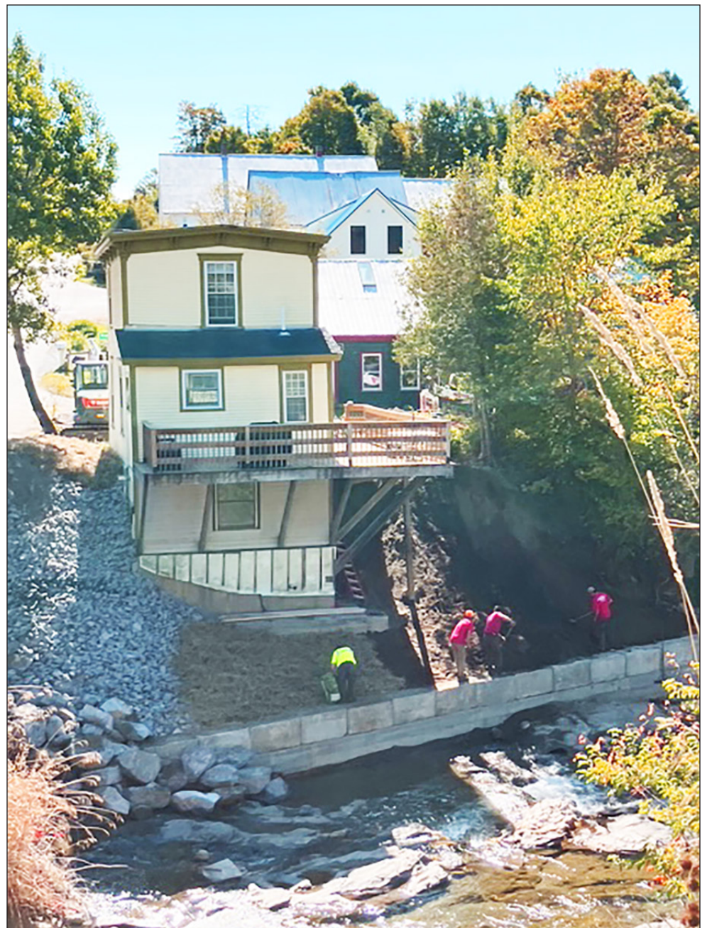
Workers with J. Merrill Construction of Middlesex complete bank stabilization and foundation work at River House on Main St. in East Hardwick earlier this month. The area was accessed with a steep ladder, with sandbagging used as needed, then a pump truck poured the concrete. The O’Brien’s expect to begin renting the property again after having to close it in 2023 following the July flood due to instability of the bank. photo by Gail O’Brien
