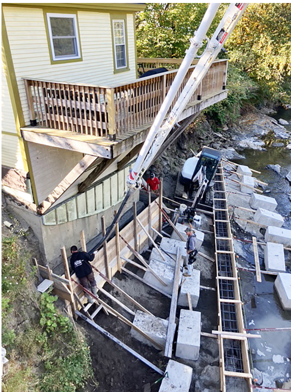
Work to stabilize the river bank at Gail and David O'Brien's River House on River St. in East Hardwick was one of three Hardwick properties approved for funding from the USDA Natural Resources Conservation Service following July 2023 flooding. New England Consulting Engineering in Morrisville developed the project, which was more complicated than the two others that were completed in 2024. A large excavator was used to drop smaller equipment down to the river by lowering it over the bank.
