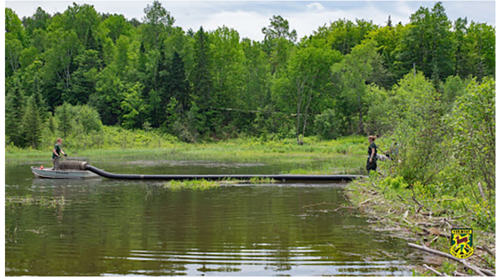
Drain pipes placed through beaver dams, with inlets a distance away, can be used to lower the level of water behind the dam, while allowing beavers to coexist there. courtesy photo
