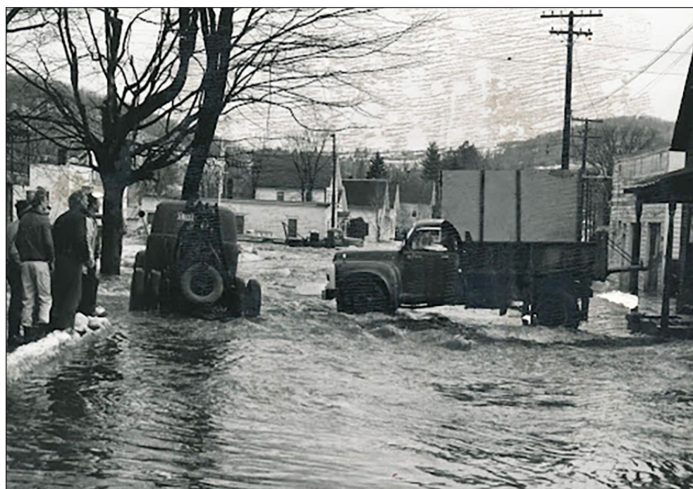
Wolcott Street near Elm Street in Hardwick, on March 5, 1964, during flooding due to a Lamoille River ice jam.
