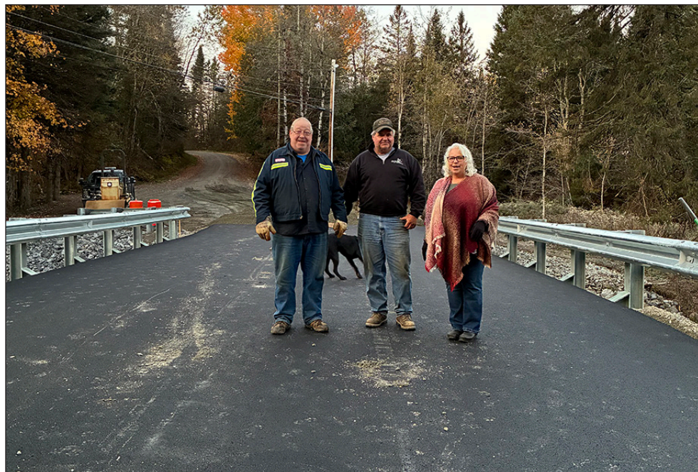
The last of Walden's flood recovery work is complete October 10 with the opening of the Orton Road bridge at its intersection with Stannard Mtn road where (from left) Walden Road Foreman Bob Bell, Austin Construction owner George Austin (bridge builder) and Walden Town Clerk Debbie Messier celebrate its opening. The bridge was destroyed in the July 10 2024 flood.
