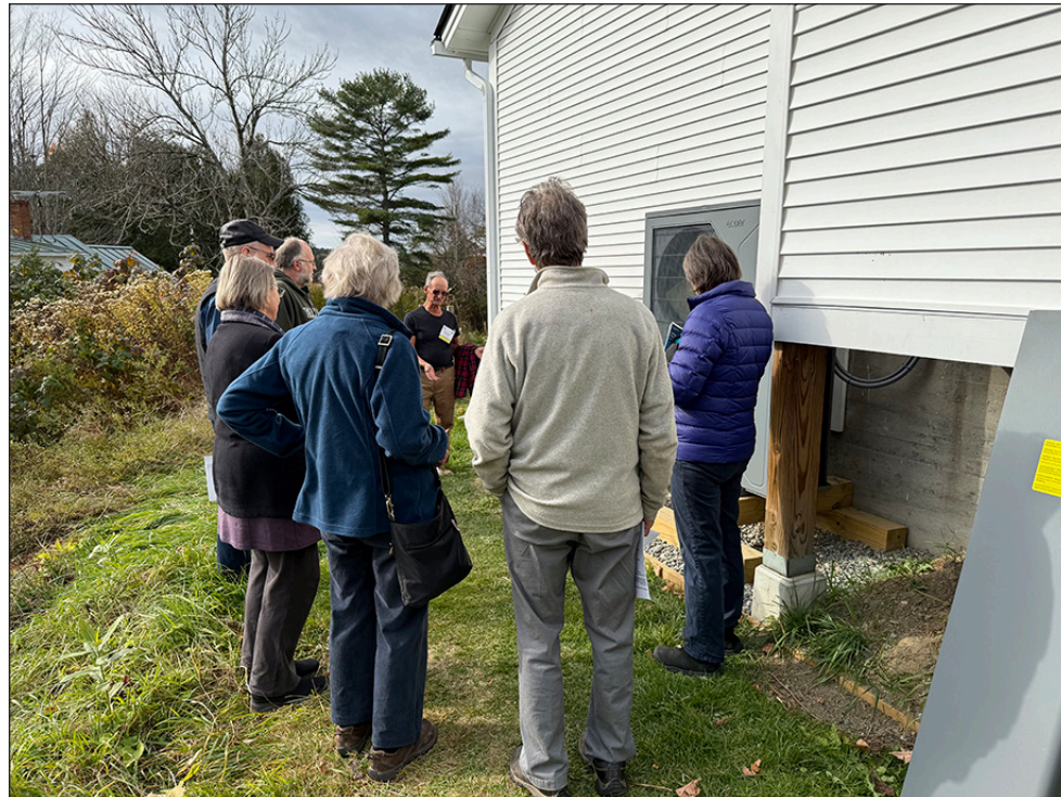
Bill Chidsey (center rear) of the Greensboro Energy & Climate Action Committee, demonstrates how the new whole building air-to-water heat pump system will work to provide energy efficient heat in the winter and cool air in the summer throughout the building. photo by Liz Steel
