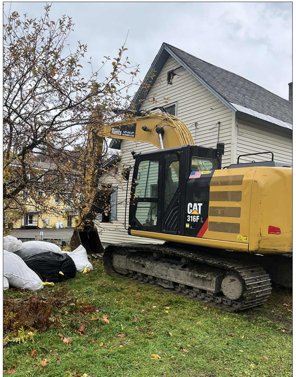
Equipment arrives at 36 Brush St. in preparation for demolition of the house and garage scheduled for Wednesday this week as a FEMA buyout following erosion of the bank of the Lamoille River on 2023 and 2024 flooding.
