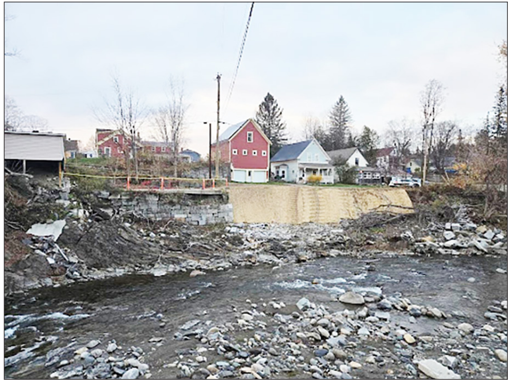
The reseeded Lamoille riverbank where a 41 Brush Street home once stood to the left of where the concrete slab of a garage is all that remains of the two Hardwick buildings removed by the state with FEMA funding. The town has hired an engineer to provide advice about next steps to protect the riverbank and area from erosion and future Lamoille River high water event.
