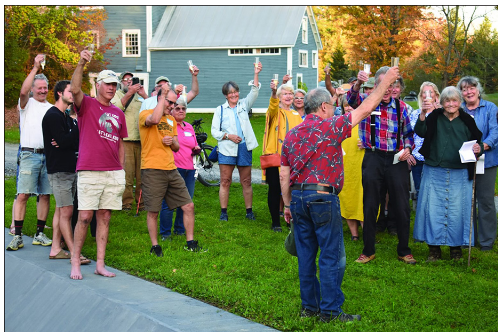
Calais state Rep. Marc Mihaly leads a toast to the newly reconstructed Curtis Pond dam in Maple Corner. photo by Mason Singer
