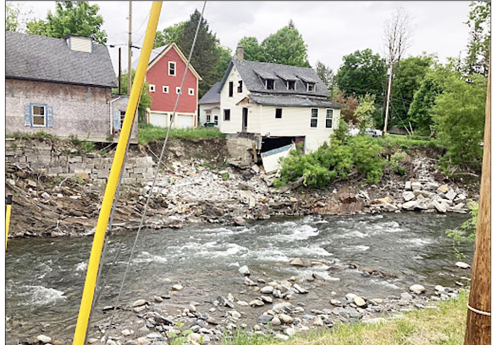
On May 29, 41 Brush Street in Hardwick had continued to be impacted by the river following repeated floods, before demolition began through the federal buyout program. photo by Kristen Leahy
