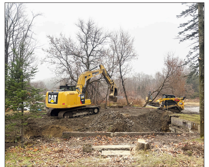
Hammond Construction uses their Cat 315S to clear out the former site of 5 Sawmill Lane in Hardwick, November 10, as part of the FEMA buyout. The state has expressed interest in a Sawmill Park on the site.
