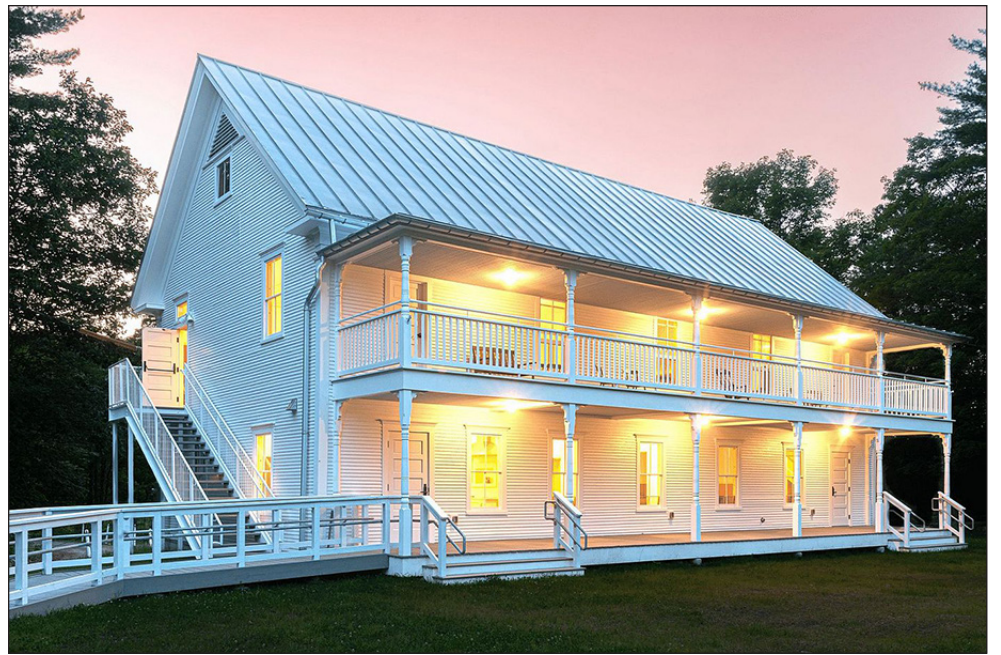
Rehabilitation of the North Calais Memorial Hall seen here, earned R. Edwards & Co. of Montpelier the American Institute of Architects Vermont Chapter 2025 Merit Award in the Historic Preservation / Adaptive Re-Use / Rehabilitation category, during its annual meeting, December 4, 2026. The architect is Ryan Edwards, AIA; general contractor is Spates Construction, Inc.; structural engineering is by Engineering Ventures, PC.
