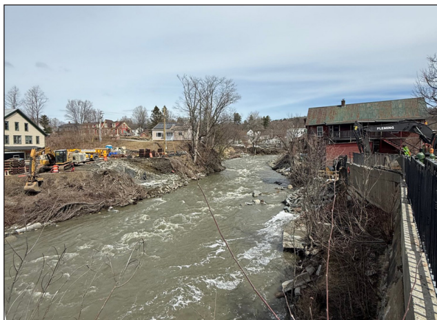
The Lamoille River work area where a new retaining wall will be built along S. Main St. to the right, with a pedestrian bridge is scheduled for installation across the river, August 7. courtesy photo
