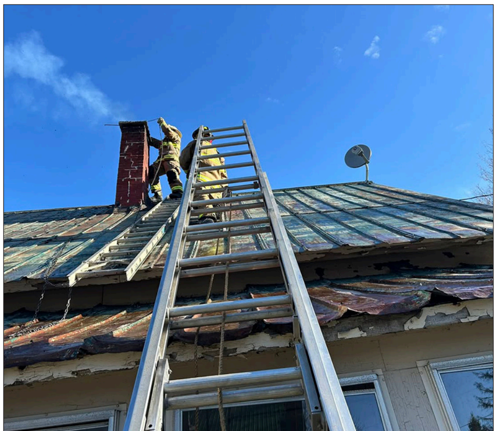
Two fire departments responded to a chimney fire on Noyestar Road, April 25. courtesy photo
