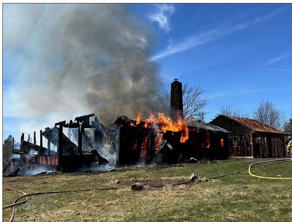
The Hardwick Fire Department joins area mutual aid partners at a controlled burn in Wolcott, April 25. The surrounding area was thoroughly sprayed down from a local pond before burning the building.
