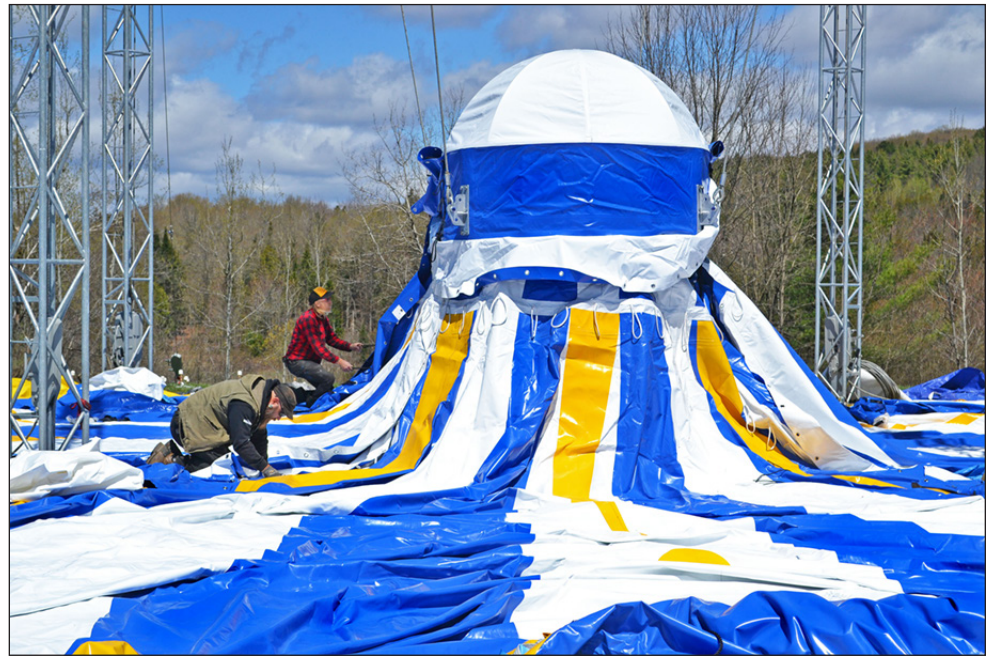
Nat Brown (left), co-owner of Crew That, a Massachusetts events logistics company specializing in tents, and Noah Pierce (right), make final connections to the cupola before it is raised. Brown worked for Circus Smirkus for 16 years as the tent boss and helped to design the new tent with Smirkus leadership. photo by Vanessa Fournier
