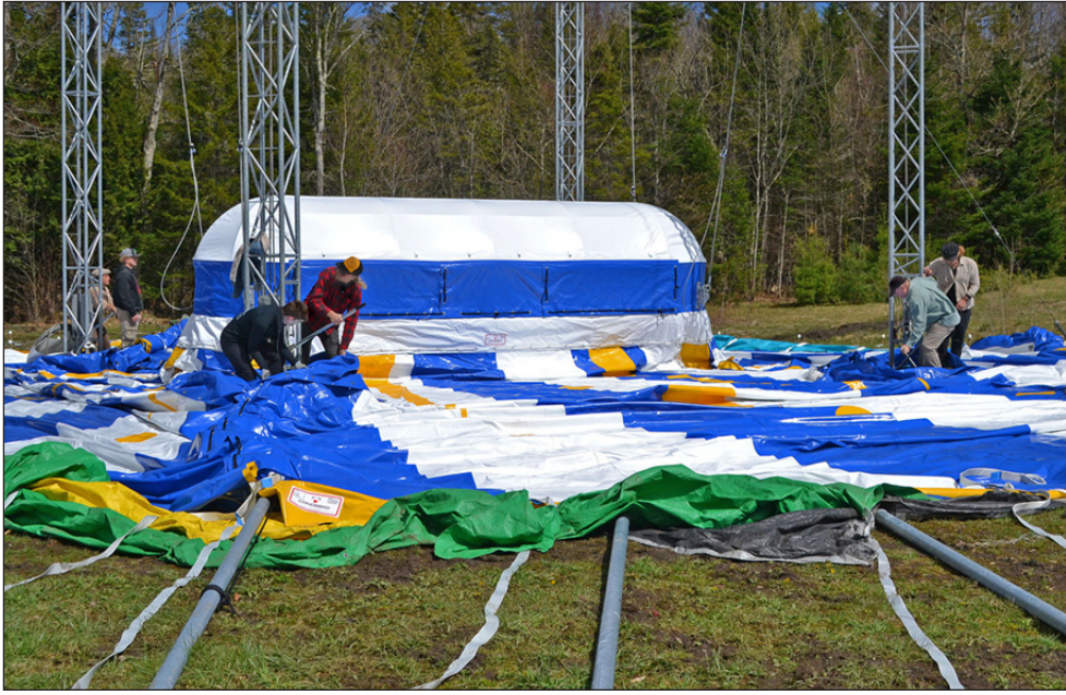
The Circus Smirkus tent crew prepare to raise the cupola after being attached to the tent canvas as the Big Top tent is raised last week for the first time. photo by Vanessa Fournier
